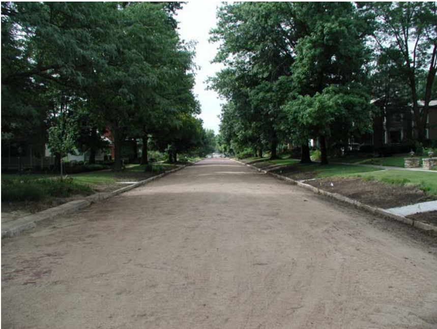
700 block looking south – sand on top of relaid bricks
