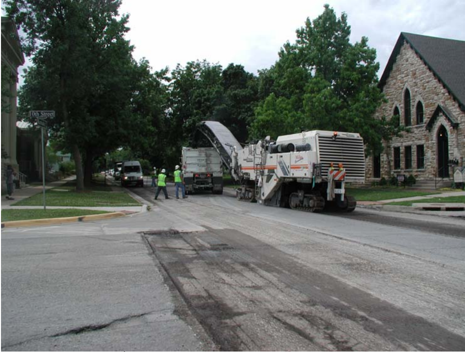
Milling operation at 10 th & Kentucky
