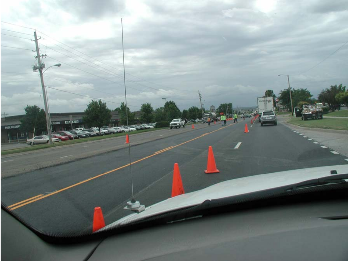
25 th & Iowa looking south – southbound lanes and center lane have been overlaid and striped
