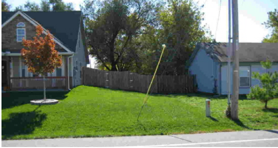
Another—where does this house drain? Onto the older neighbor, of course. Strange as this may seem, the City of Lawrence building codes not only allow but encourage this practice.
