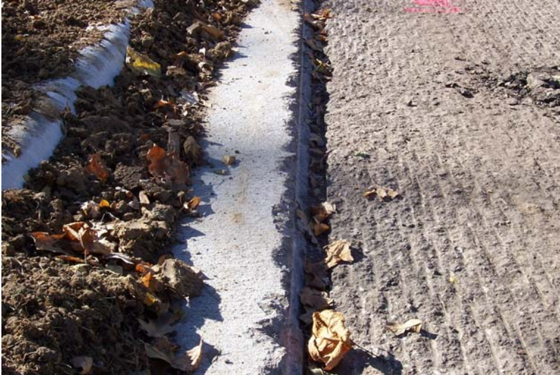
Edge of new curb & gutter damaged by milling machine is vulnerable to more rapid deterioration.
