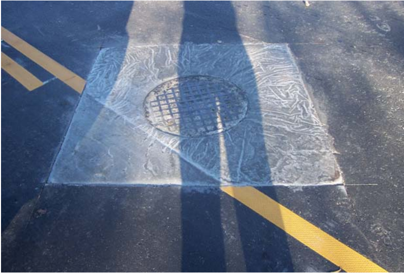
Concrete slab around manhole has imprints of creases in plastic sheeting used for protection from weather. (Example of aesthetic rather than functional issue.)
