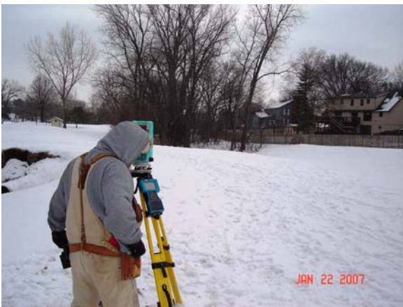
Surveying pipe alignment on the golf course
