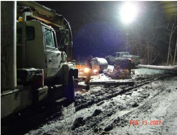
Pipe reaming at night on the AGC
