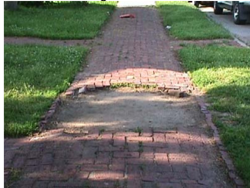
Bricks missing, trip hazards
