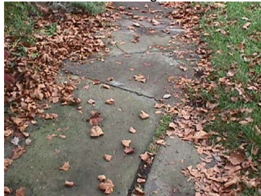
Slate walk with concrete patch
