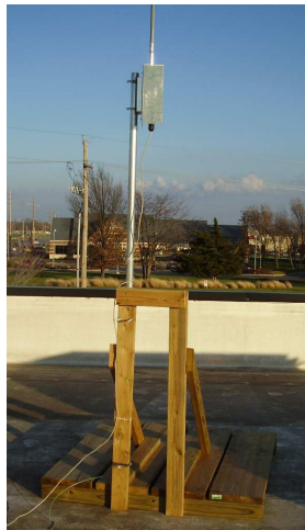
Figure 1: Example of Non-Penetrating Roof Mount Installation
