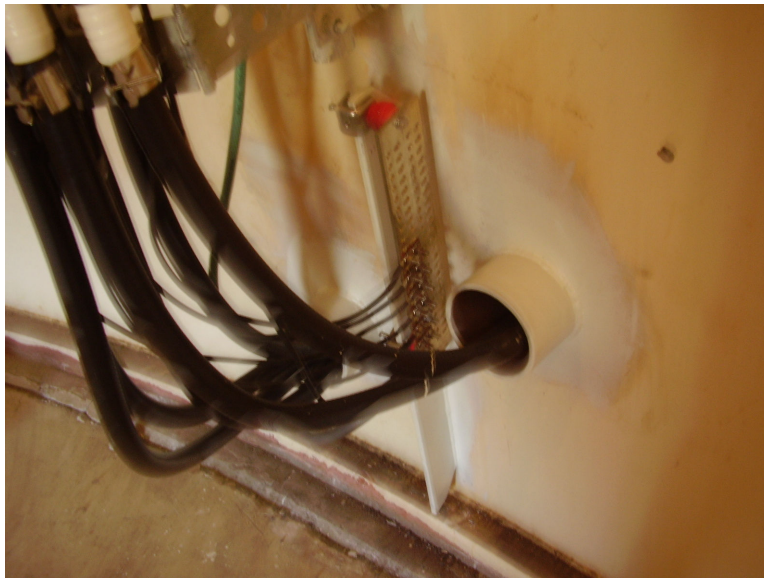
Cable entry point inside Tower
