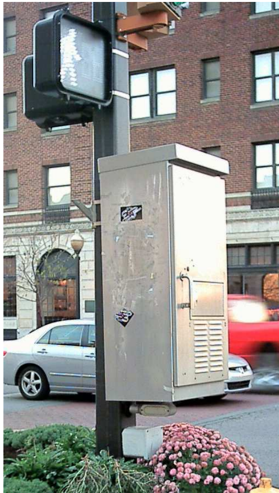
Figure 5 Large Nema Enclosure at 7th & Mass
