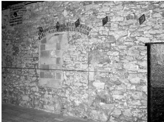
Existing brick and stone masonry - Zone 1
