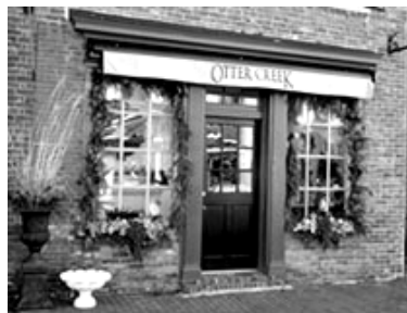
The infill storefront in the building above creates the false impression of an original retail store rather than the historical industrial use of the building
