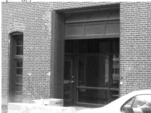
Original door opening is retained. The new infill incorporates an entrance and half "closed" garage door as well as transparent glazing is an appropriate treatment where there is no documentation of the original door.
