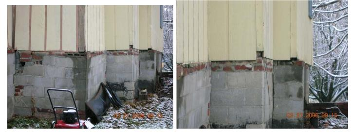
Rear porch – rotted, deteriorated/damaged foundation and supports:
