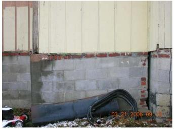
Deteriorated foundation, south wall:
