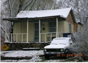
Front porch, rotted porch structure, flooring and roof:
