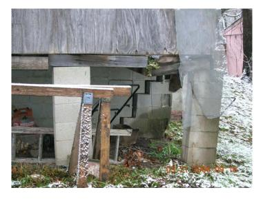
North side, view from rear: (rotted roof, open crawl space)
