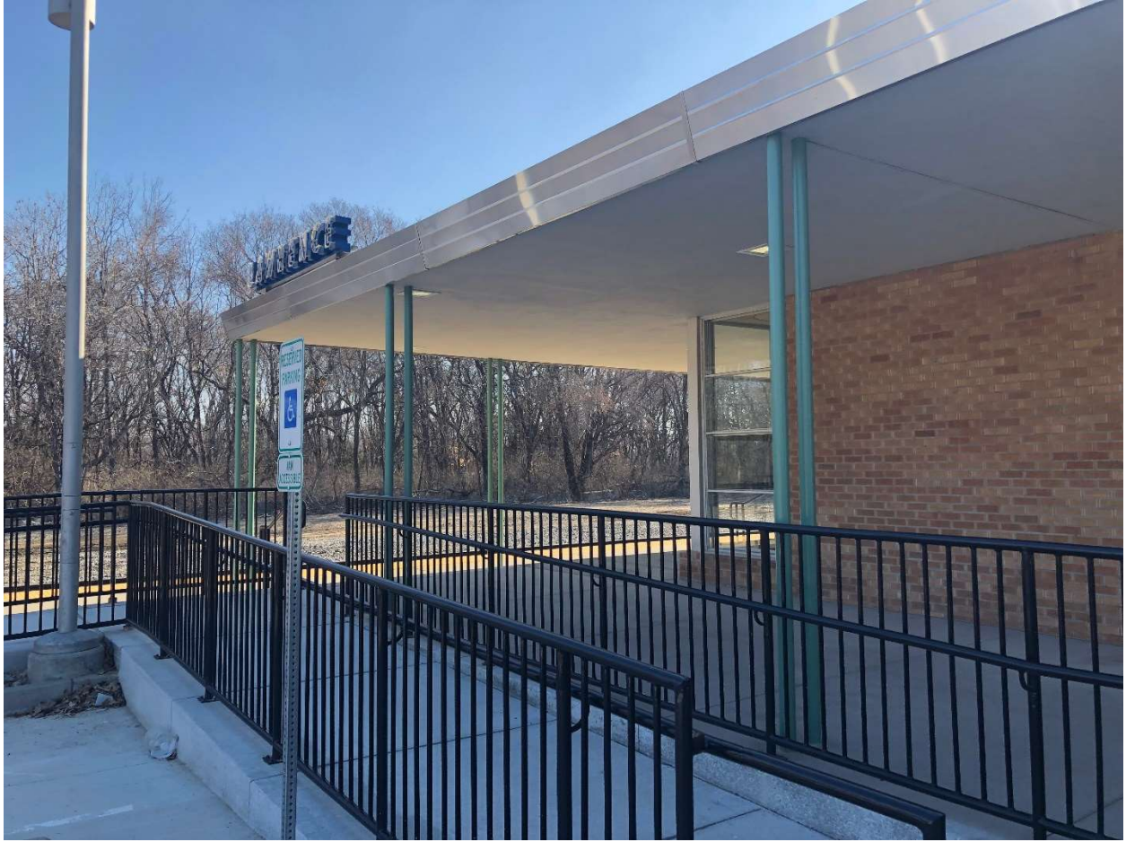
Exterior West side
